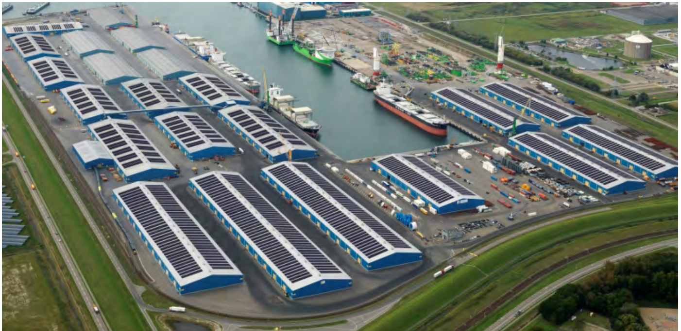
Verbrugge International 25 Million kWh rooftop solar project 19
