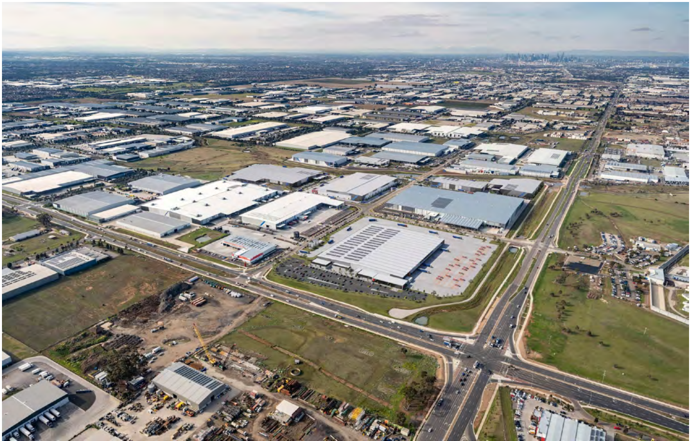
Charter Hall's Midwest Logistics Hub (Truganina, Australia), 2MW installed solar capacity
